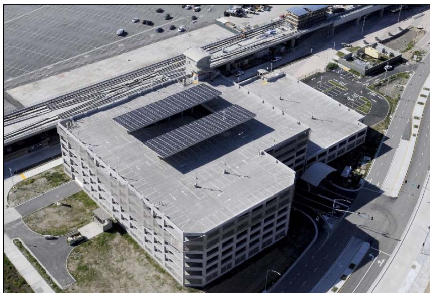
Berryessa Station Parking Garage Solar Panel System
