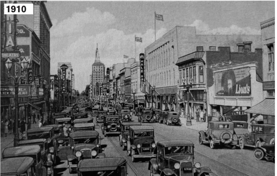
View from First Street, one of the main retail streets in San José.
