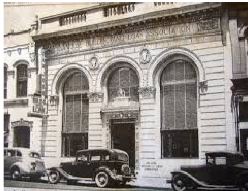
Fig. 3-49 Historic San Jose Building and Loan Association Building 2019 (Top) and 1930 (Bottom)
