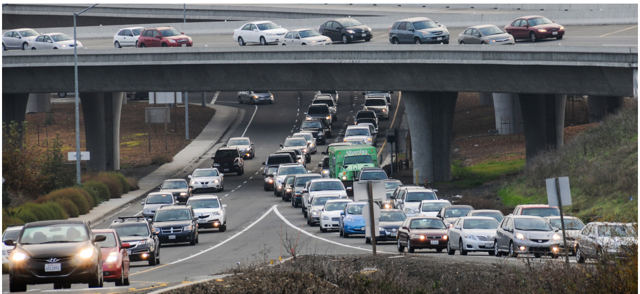
Highways require a lot of maintenance.
