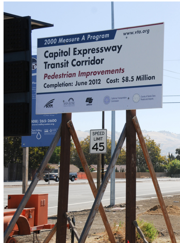
Walkways require maintenance and improvements.
