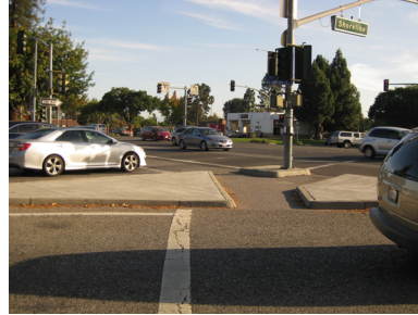
Wide curb radii and underbuilt porkchop at intersections
