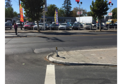
Incomplete pedestrian facilities at 1st/2nd Streets
