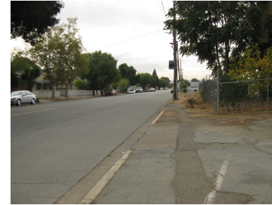
Missing sidewalks within Focus Area
