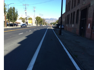
Missing sidewalks along Keyes St
