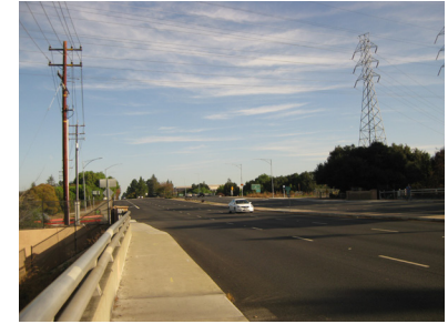
Narrow sidewalks on the SR 85 overcrossing
