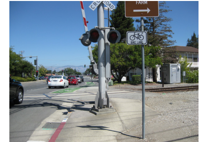
Inconsistent and unclear pedestrian walkway at rail crossing.
