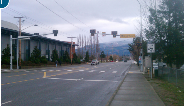
Pedestrian Hybrid Beacon (High Intensity Actuated Crosswalk, or HAWK Signal)
