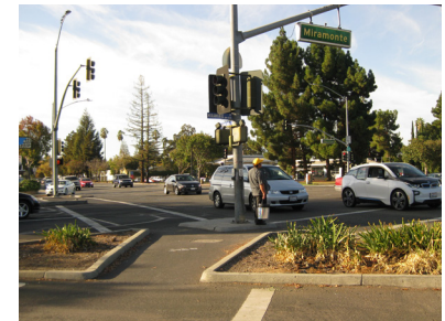
Existing pedestrian crossing improvements at Shoreline Blvd-Miramonte Ave/El Camino Real
