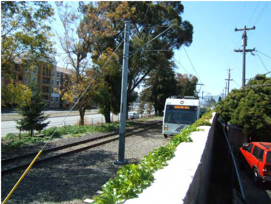
FIGURE 13 - SITE 4 LOOKING SOUTH FROM BARRIER WALL WITH REVENUE TRAIN TRAVELING NB ON SINGLE TRACK
