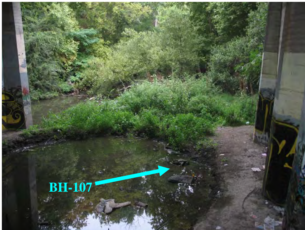
Figure 3 – Photo of Planned BH-107 Location Below Coyote Creek Bridge, looking northwest, Pier No. 3 on the right. Photo shows vegetation prior to work.
