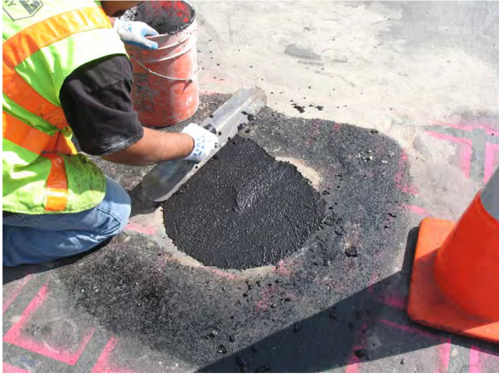
Figure 16 – Photo of Installed Patch. BASF Set 45 material had limited workability.
