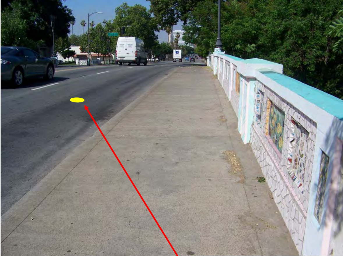
Figure 6 of 8. View looking westbound at Santa Clara Street bridge deck surface.
