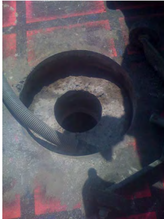
Figure 10 – Photo of Completed Core Hole Through Bridge Deck
