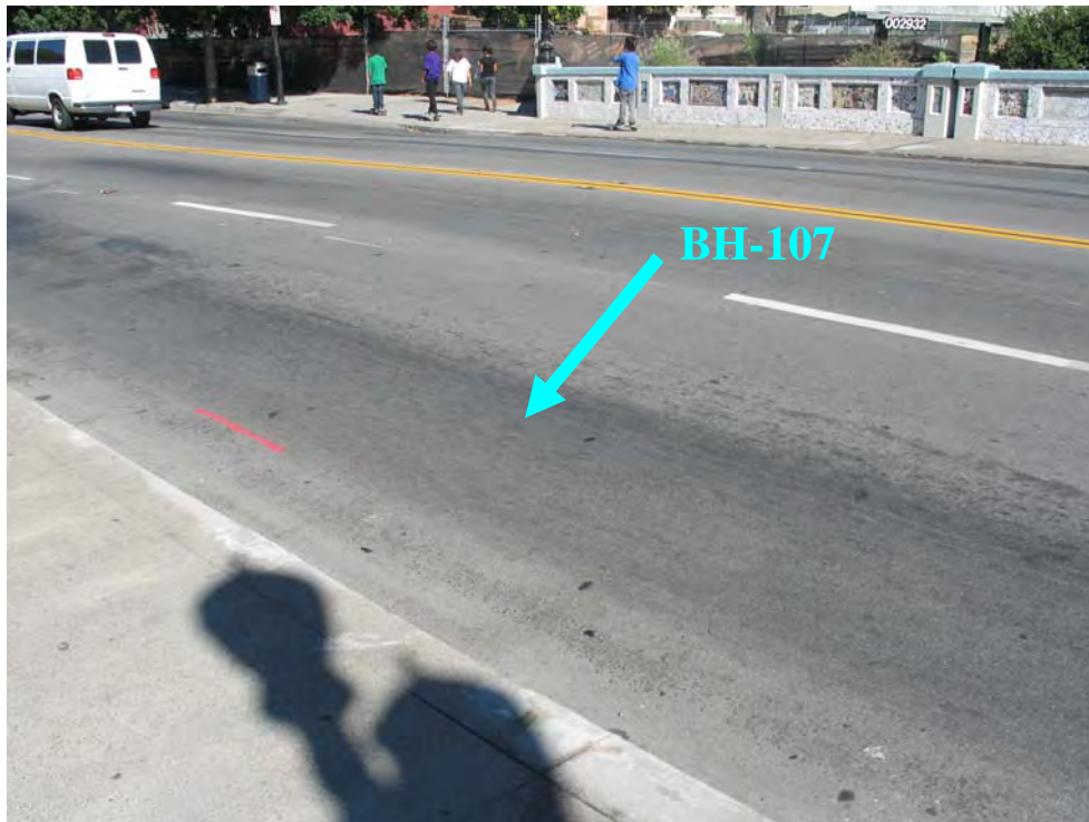
Figure 2 – Photo of Planned BH-107 Location on Coyote Creek Bridge, Looking Southeast from north sidewalk, south end of Pier No. 3 located at joint in south guardrail.
