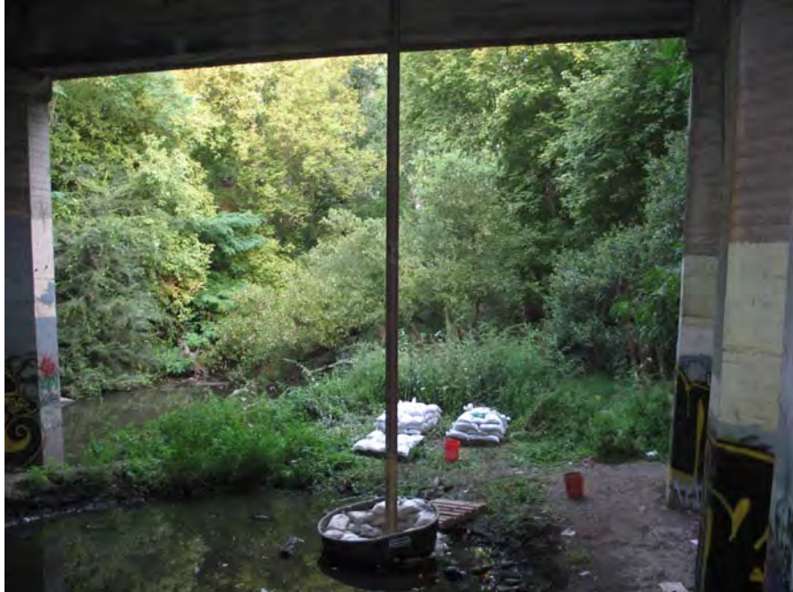
Figure 12 – Photo of Conductor Casing and Isolation Tub with Sandbags at Ground Surface. Pier No. 3 is on the right, Pier No. 2 on the left. The photo is looking northwest.
