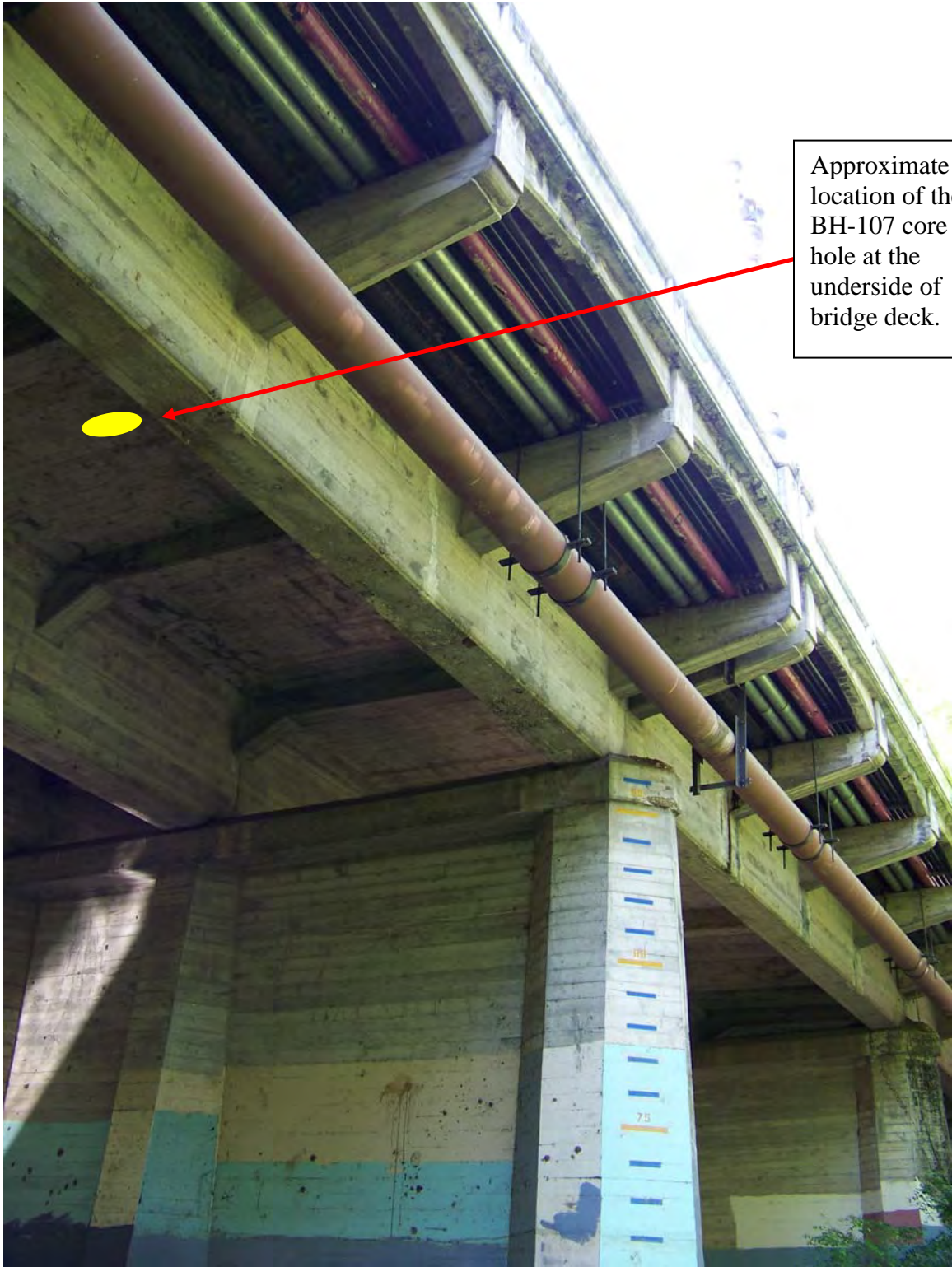
Figure 7 of 8. View from underside of bridge deck.
