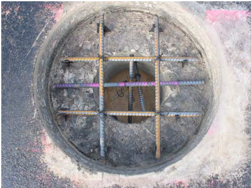
Figure 15 – Photo of Patch Reinforcement. Form board is shown below core hole.
