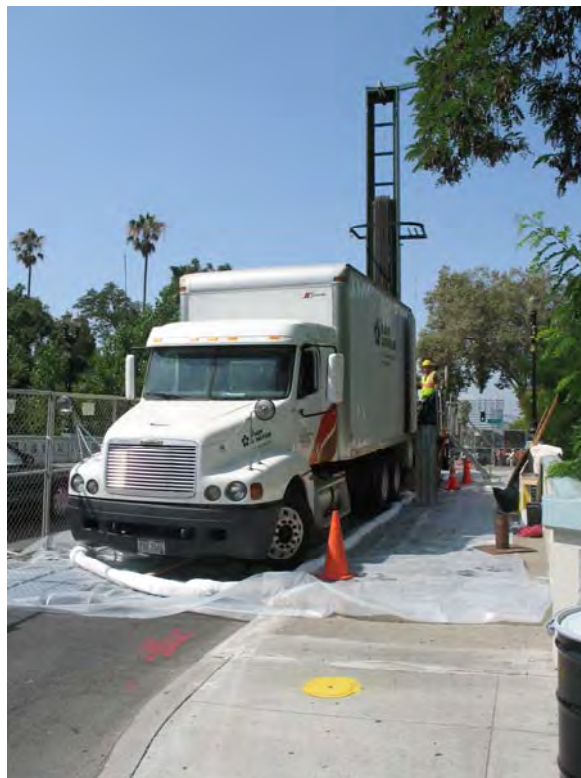
Figure 13 – Photo of Drilling Operation on Bridge Deck. Photo is looking southwest.
