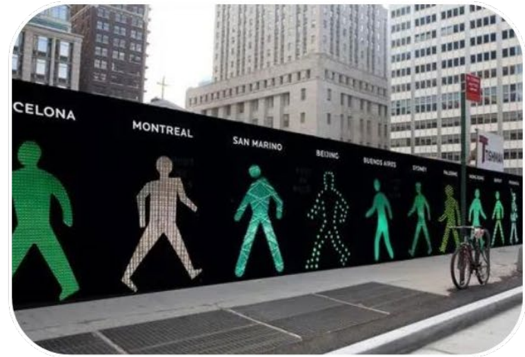
Install and maintain graphic panels along construction staging areas
