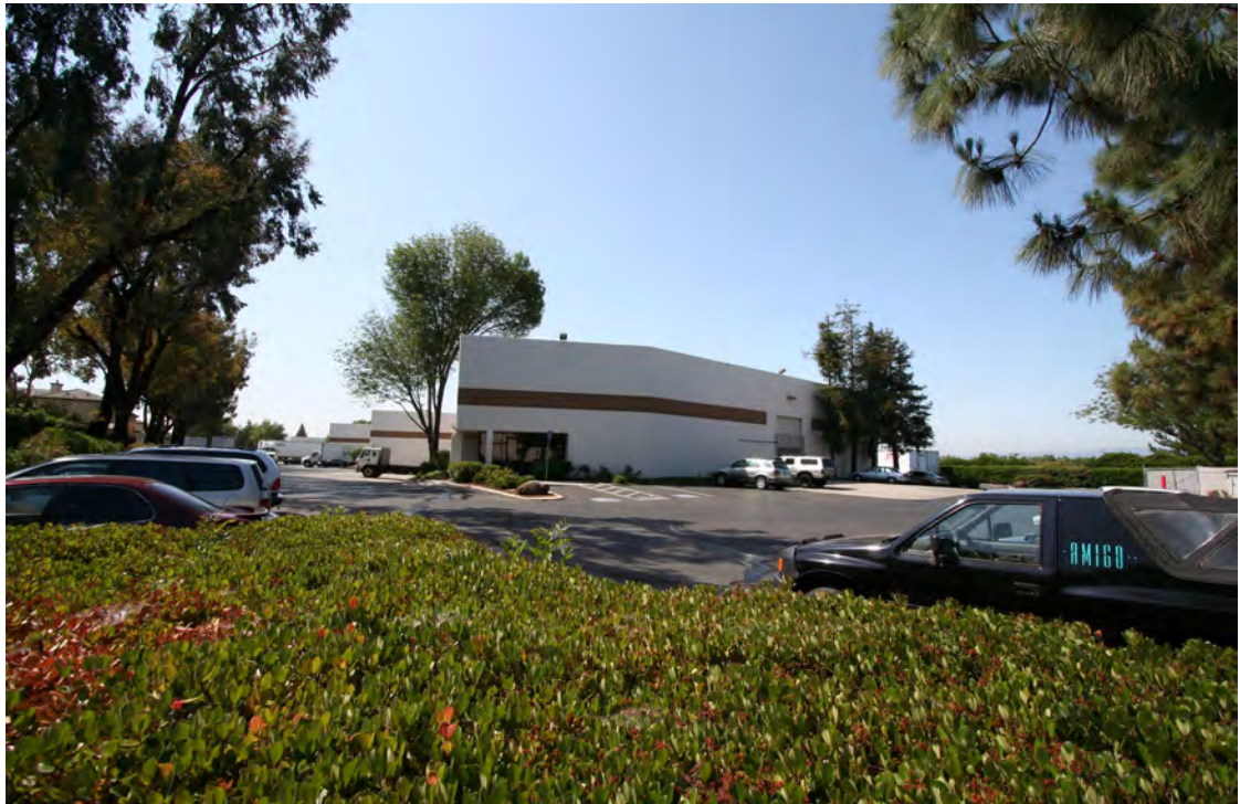
Existing View of Berryessa Station South Option Location (view to the southwest from the end of Salamoni Court)
