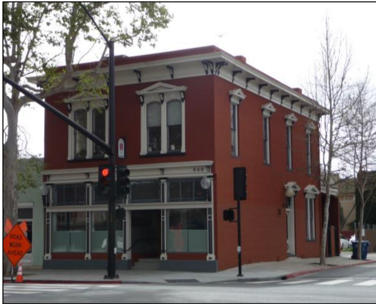
Photograph 4-21: Commercial building at 848 The Alameda.
