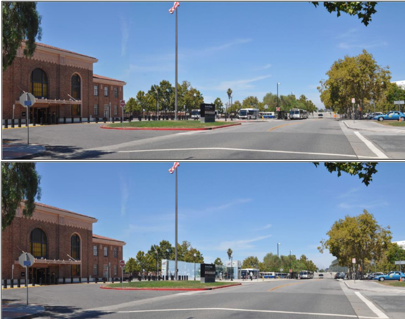
Figure 5-13: Existing View (top) and Simulated View (bottom) of the Diridon Station South Option E1 station entrance option looking north along Cahill Street showing the Southern Pacific Depot (left).
