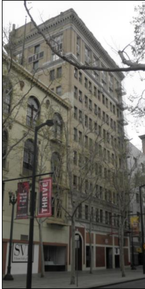
Photograph 4-11: The Commercial Building (22 North 1 st Street).
