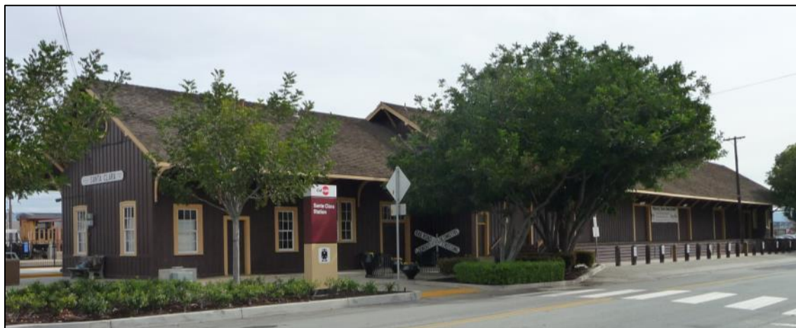
Photograph 4-24: Santa Clara Station (1 Railroad Avenue).
