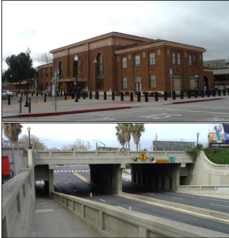
Photographs 4-19 and 4-20: Cahill/Diridon Station (top) and Santa Clara/Alameda Underpass (bottom).
