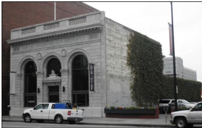
Photograph 4-13: San Jose Building and Loan (81 West Santa Clara Street).
