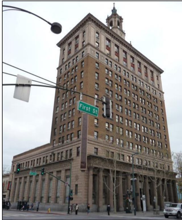
Photograph 4-9: The Bank of America building at 8-14 South 1 st Street.
