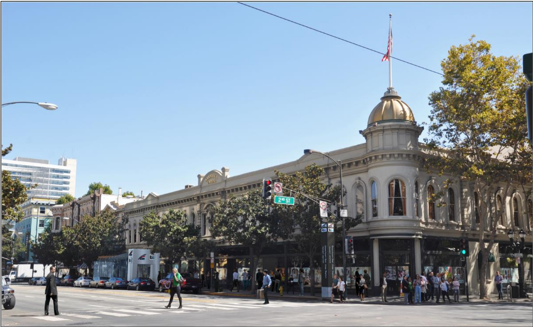
Figure 5-5: San Jose Downtown Commercial District, Existing View (top) and Simulated View (bottom) of the Downtown San Jose Station—East Option E1 entrance option. Views are looking southeast along Santa Clara Street showing South 3 rd Street (far right) and historic district contributor (Map Reference E-13, middle right, and Map Reference E-14, middle left).
