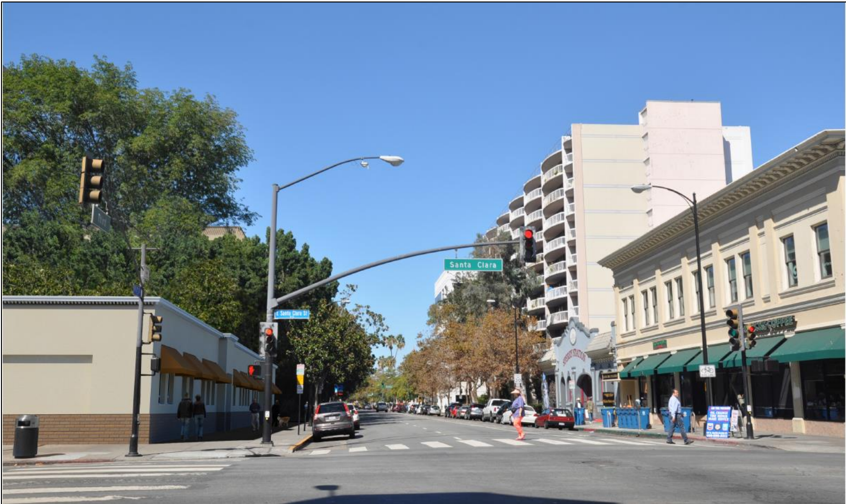
Figure 5-11: The Sperry Building (30 North 1 st Street), Existing View (top) and Simulated View (bottom) for the Downtown San Jose Station—East Option, facing northeast on North 1 st Street.
