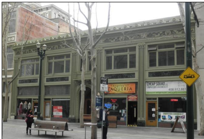
Photograph 4-10: Detail of west side of the Realty Building's main façade (19 North 2 nd Street).
