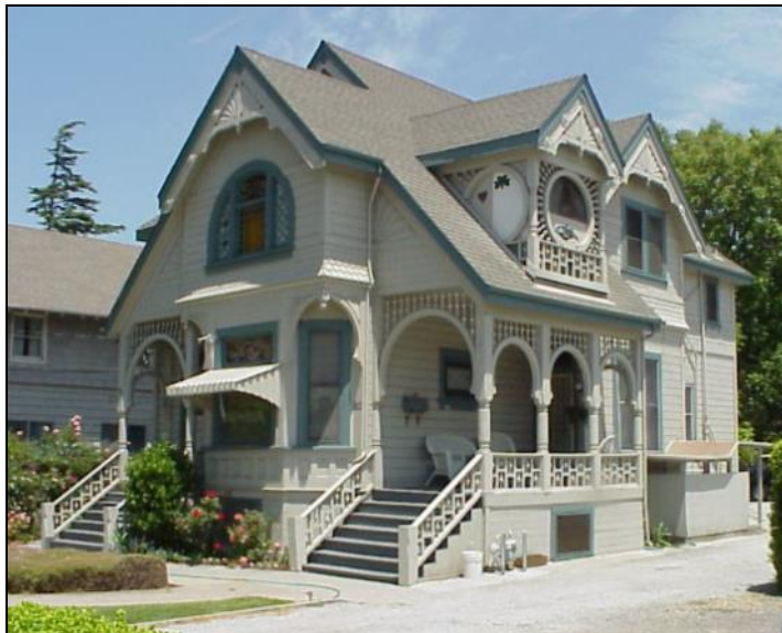
Photograph 4-22: Residence at 176 North Morrison Avenue.
