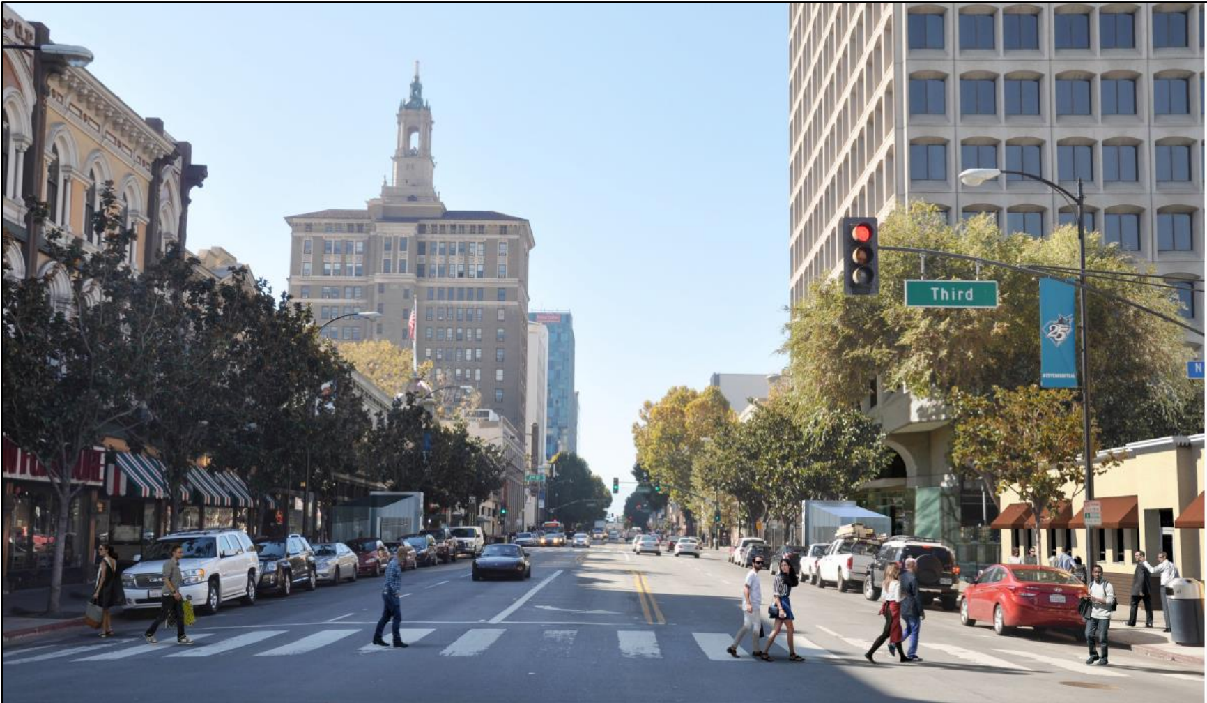
Figure 5-4: San Jose Downtown Commercial District, Existing View (top) and Simulated View (bottom) of the Downtown San Jose Station—East Option E1 entrance option. Views are looking southwest along Santa Clara Street showing historic district contributors (Map Reference E-13) at left.
