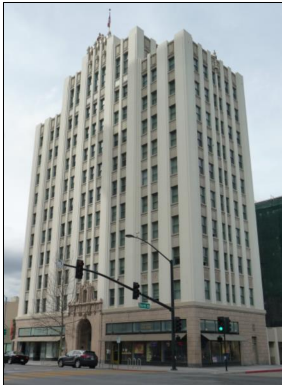
Photograph 4-5: Vintage Towers (Medico Dental Building) at 227-247 East Santa Clara Street.
