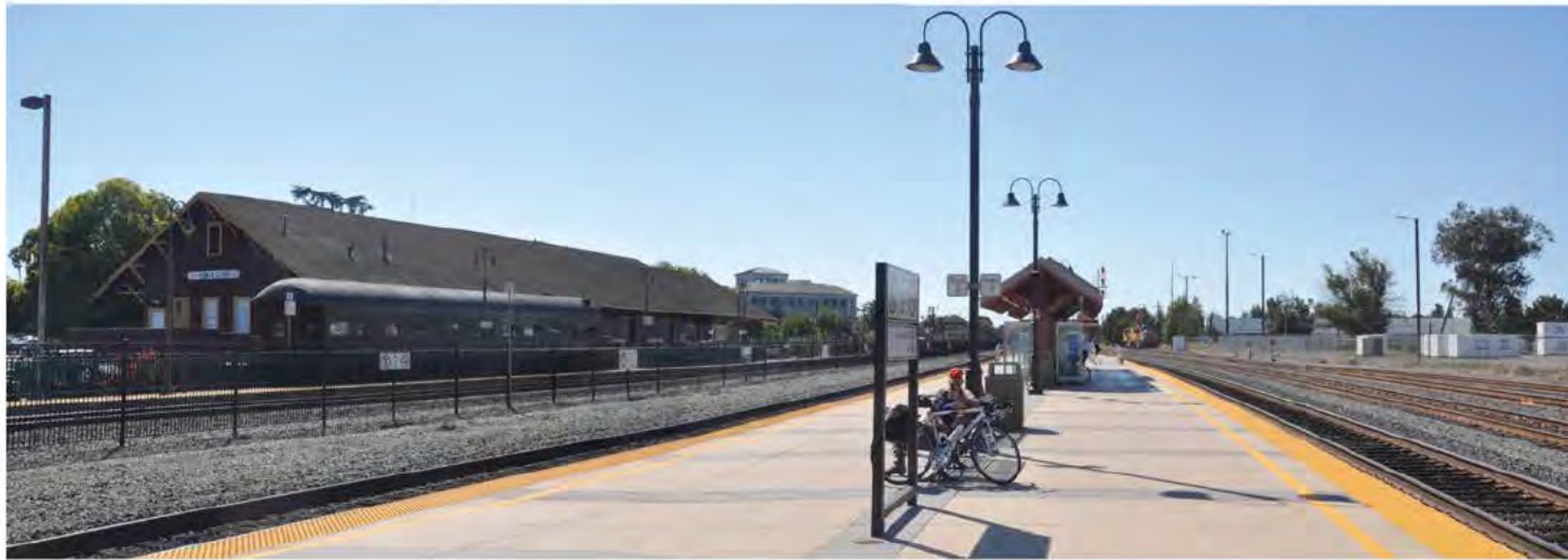
Existing view of the Santa Clara Caltrain Station and Platform (view to the northwest from the Santa Clara Caltrain Station platform)
