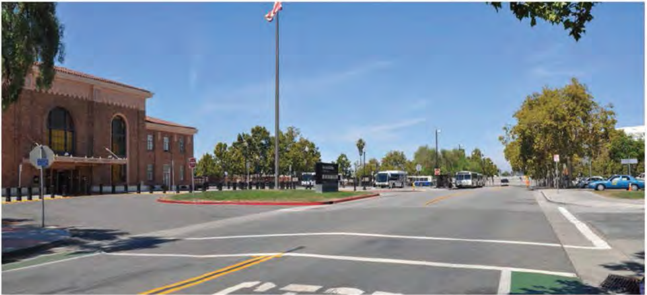
Existing view of the Diridon Caltrain Station (view to the northwest from Cahill Street)
