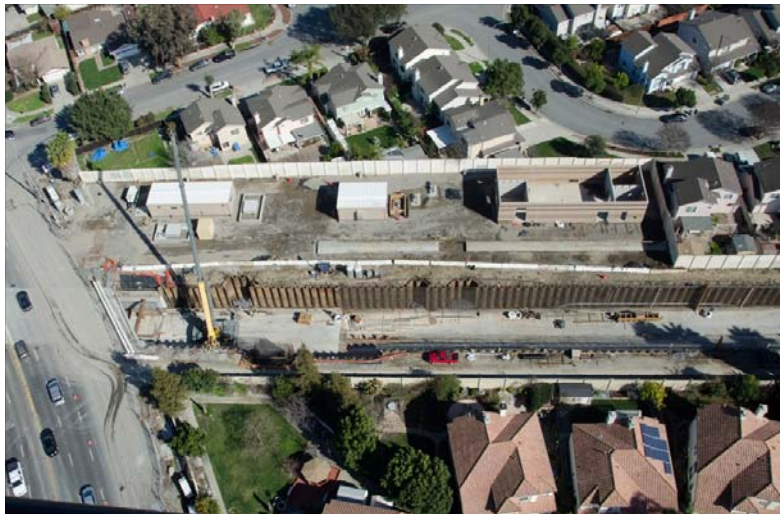
Trench at Hostetter Road with systems facility adjacent to alignment
