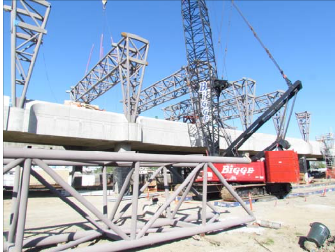
Berryessa Station canopy
