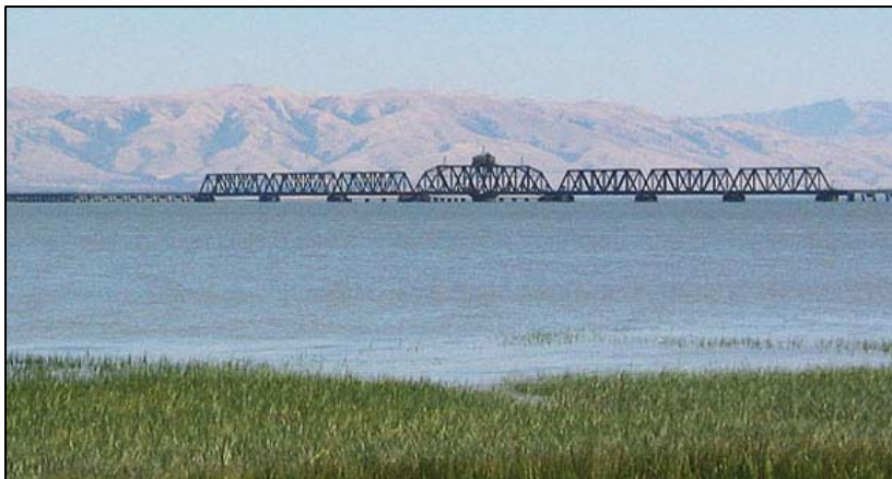
View of Dumbarton Bridge from the West
