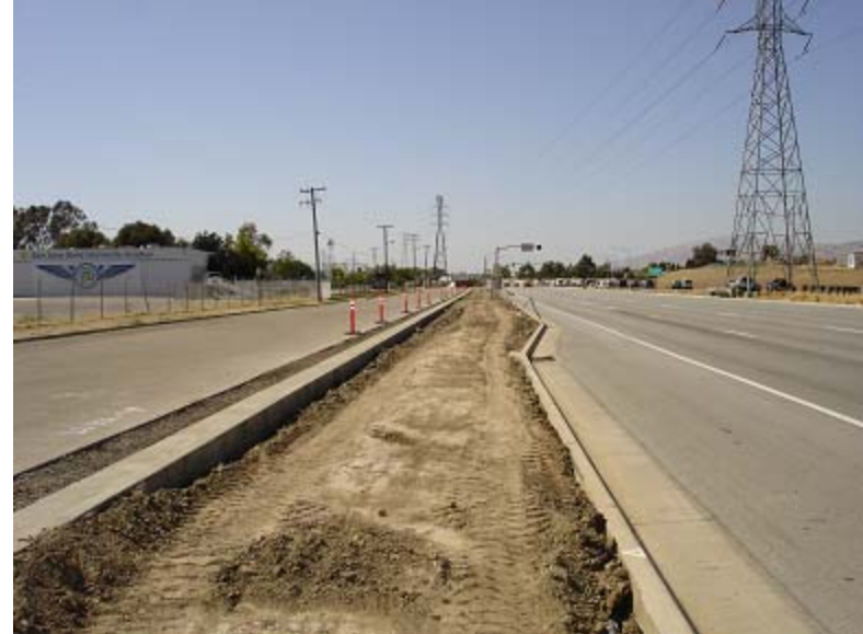
Grading for sidewalk near Cunningham Park
