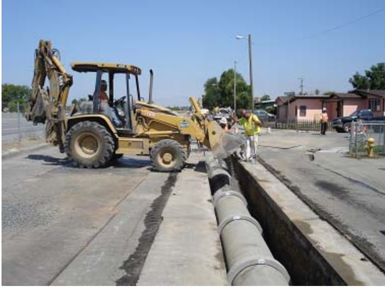
Storm Drain Relocation along Capitol Avenue
