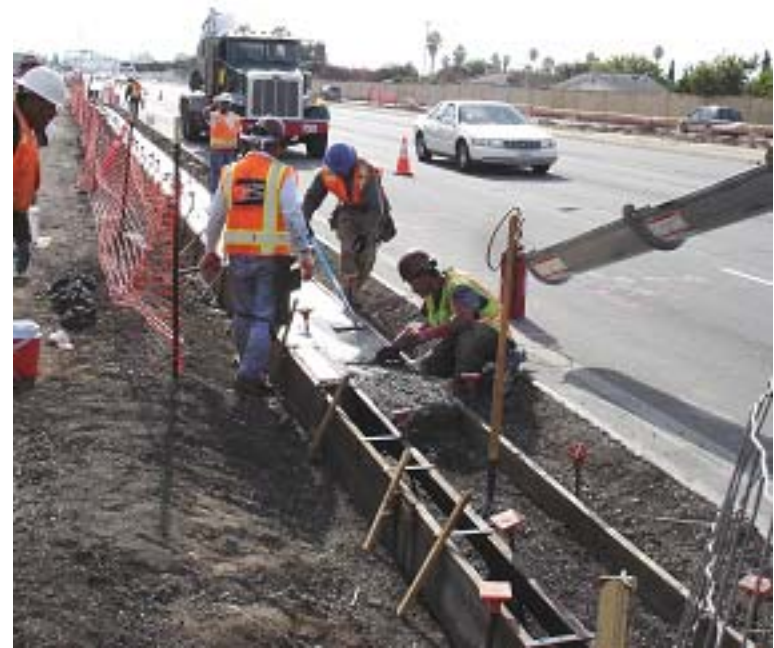
Forming new curb and gutter south of Story Road
