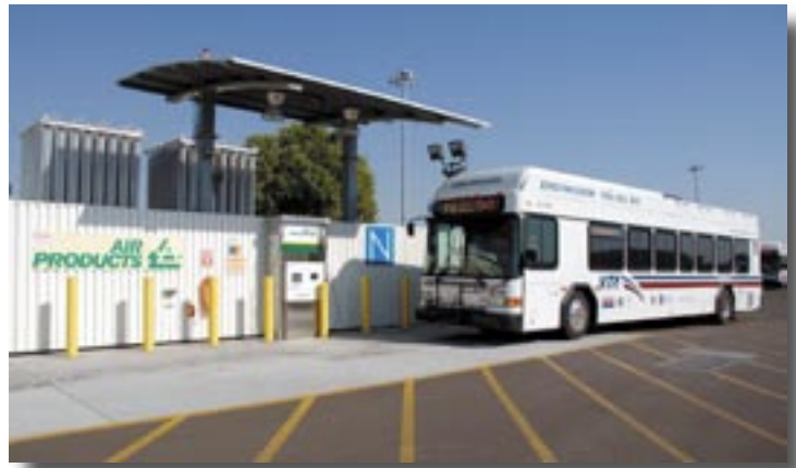
Zero-emission bus at hydrogen fueling facility
