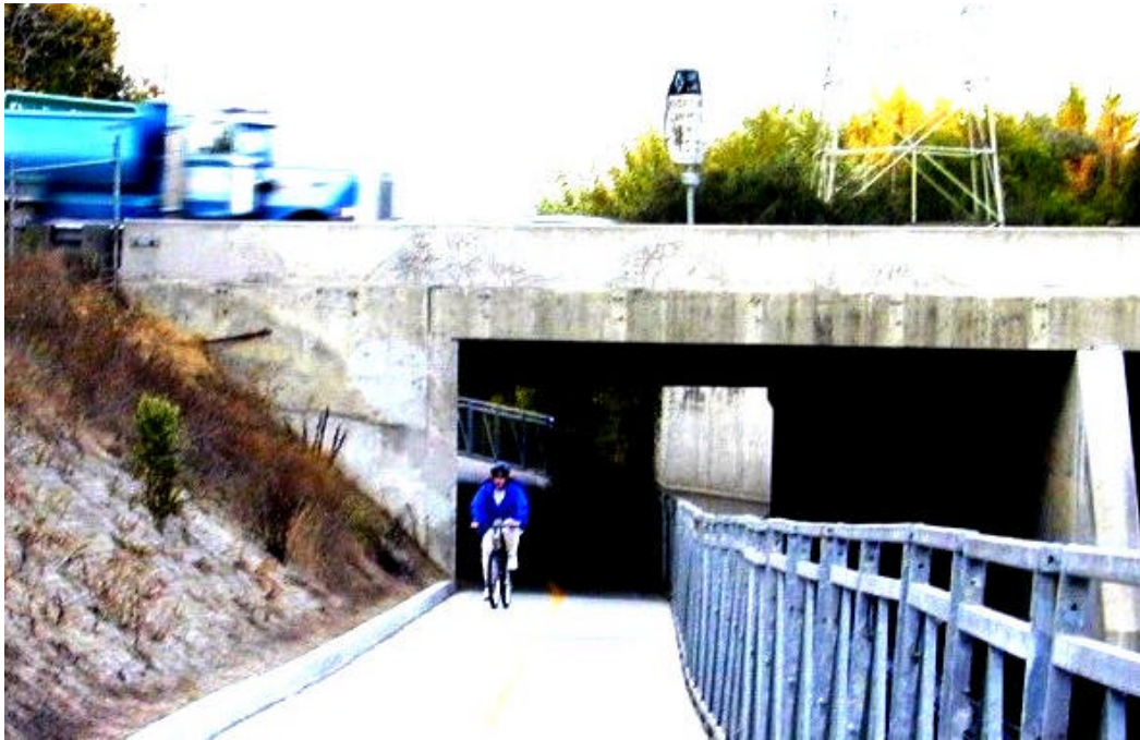
Figure 2-3 Stevens Creek Trail undercrossing at US-101
