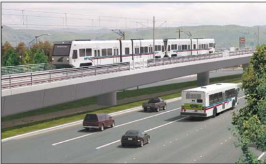
Example of elevated LRT track way. Some of the new light rail line may need to be elevated in an "aerial" configuration.
