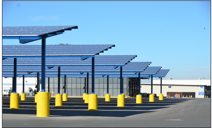
Shade and weather protection are provided for buses at VTA's Cerone Maintenance Division, 3990 Zanker Road in San Jose.
