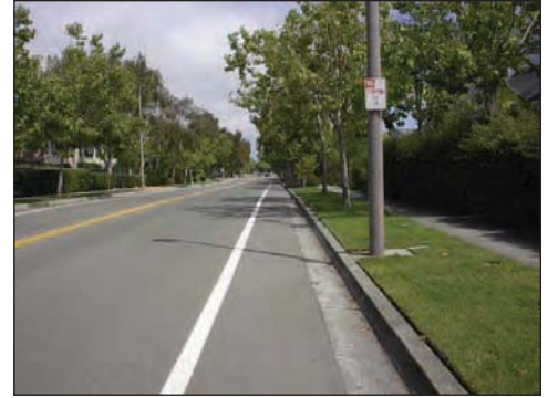
Bike lane-parking prohibited.
