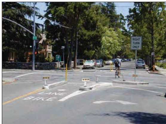
Bryant Street at Embarcadero Road in Palo Alto, where bikes may proceed straight but motor vehicles must turn right.
