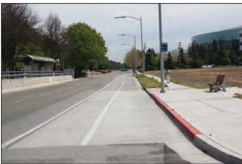
Concrete bus pad on N. First Street, San Jose.
