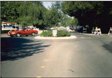
Residential traffic circles at two intersections.
