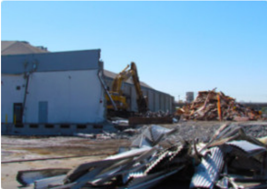
Construction has started on the new Milpitas BART Station. Credit BART
