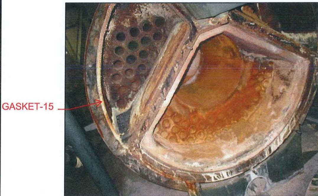
Photograph 8: Boiler Insulation Sampling
