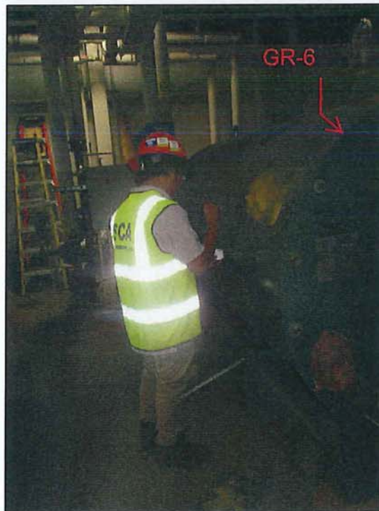
Photograph 4: Boiler Insulation Sampling
