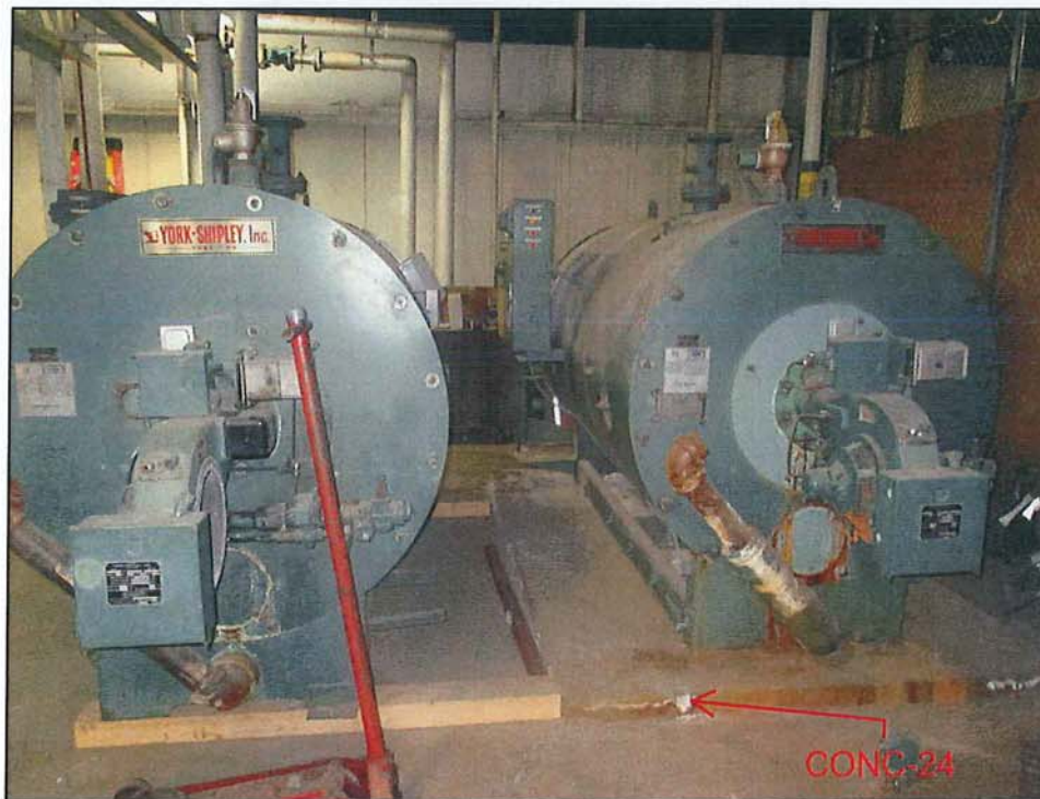
Photograph 18: Boiler Gray Concrete Pads.
