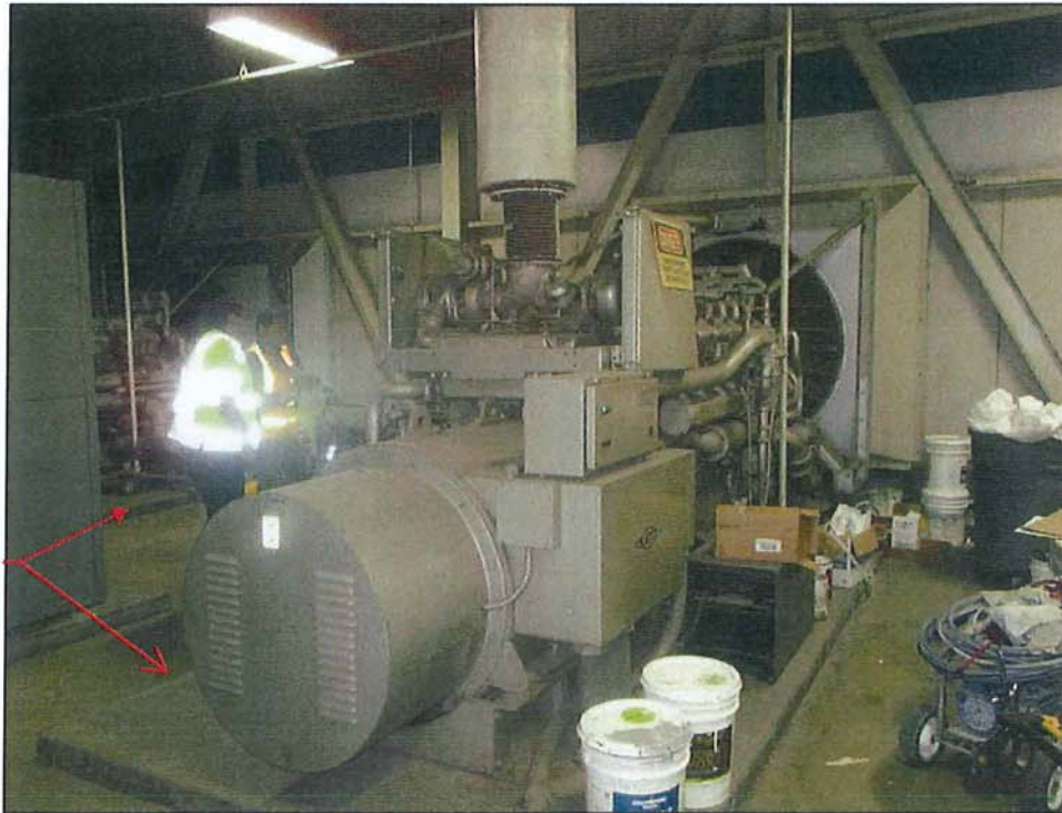
Photograph 19: Gray Concrete Pads- Diesel Generators
