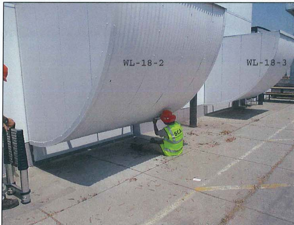
Photograph 2: Exterior Dampers: Exterior Samples WL-18-2 & WL-18-3
