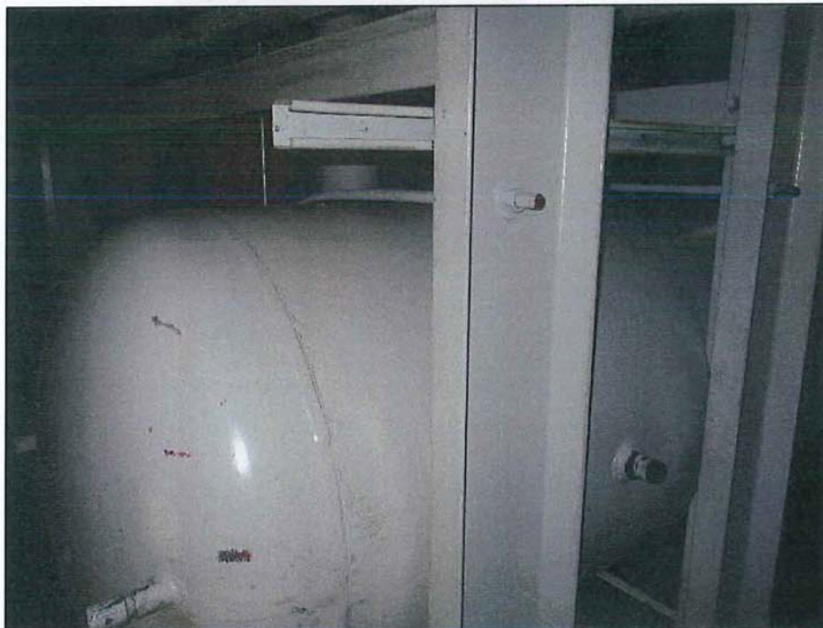
Photograph 10: Expansion Tanks/Brackets
