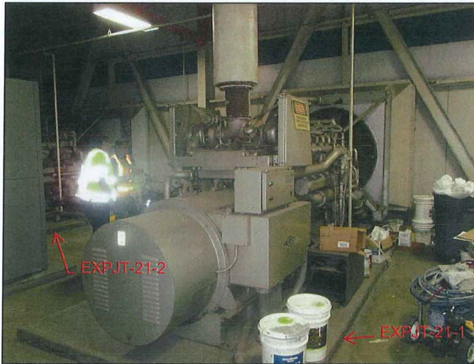
Photo 17: Expansion Joints Caulking
