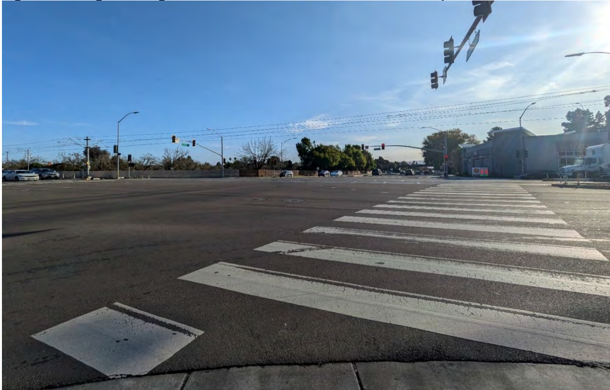
Figure 23. Long Crossing Distances at Hostetter Road and North Capitol Avenue Intersection
