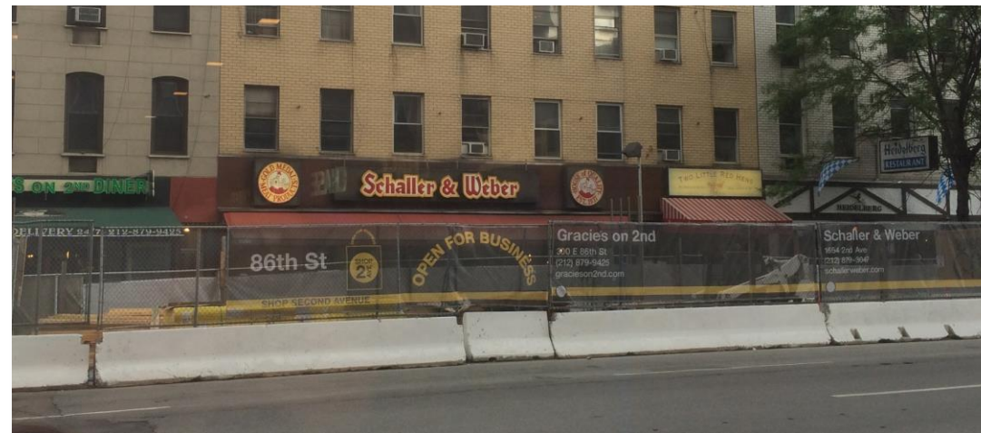
"Open for Business" signage during construction of 2nd Avenue Subway in New York
