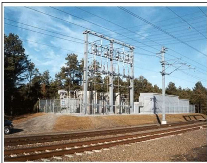
Example Traction Power Substation
