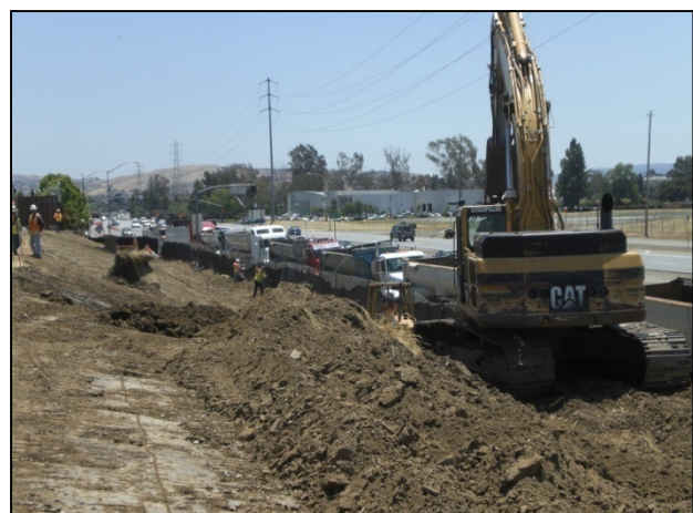
Excavation at Capitol Expressway
