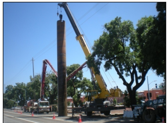
Blossom Hill Cast In Drilled Hole (CIDH) Foundation for Bridge Bent 2
