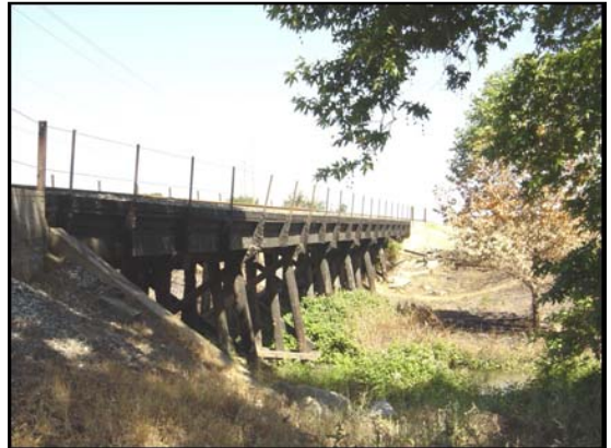
Llagas Creek Bridge
