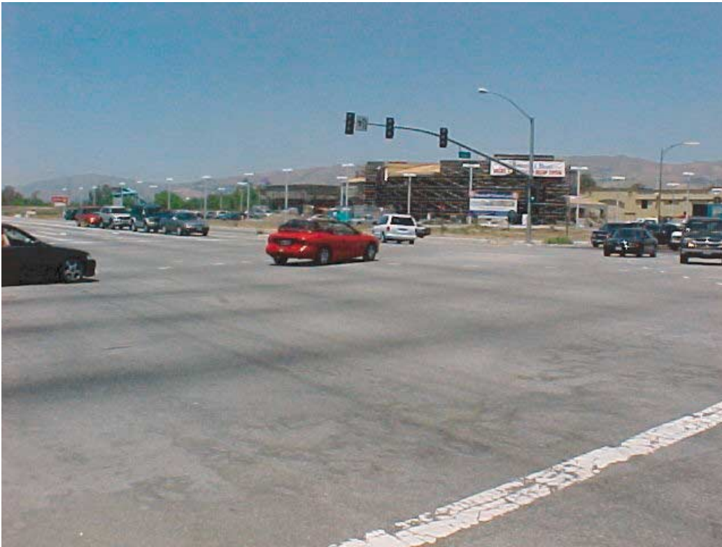
Figure 4.18-11b Views of construction at Tully Road/Capitol Expressway.
