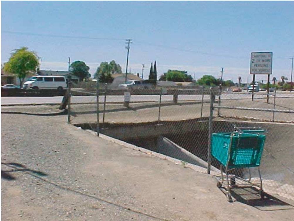
Figure 4.18-5a Existing view of Silver Creek overcrossing at Mervyn's Way.
