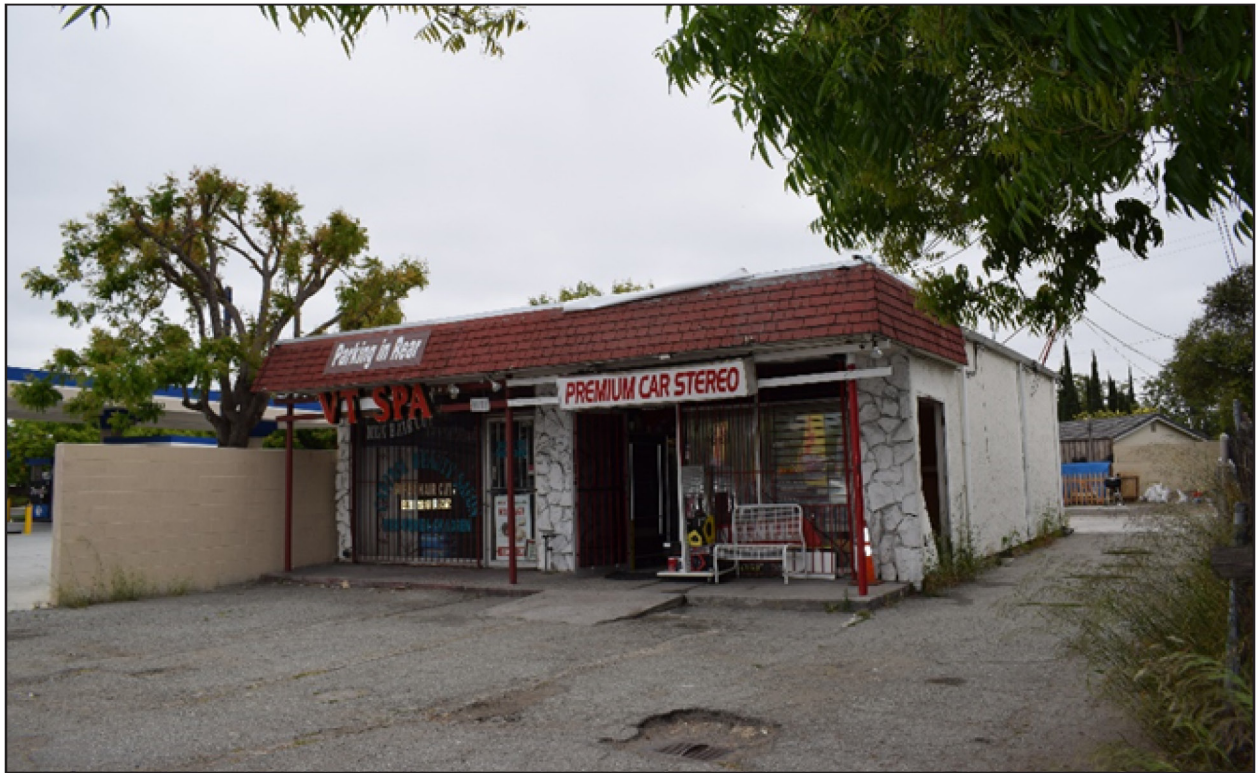
a. View of the building at 1091-1093 S. Capitol Avenue.
