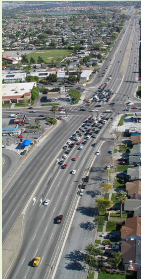
Existing Story Road
