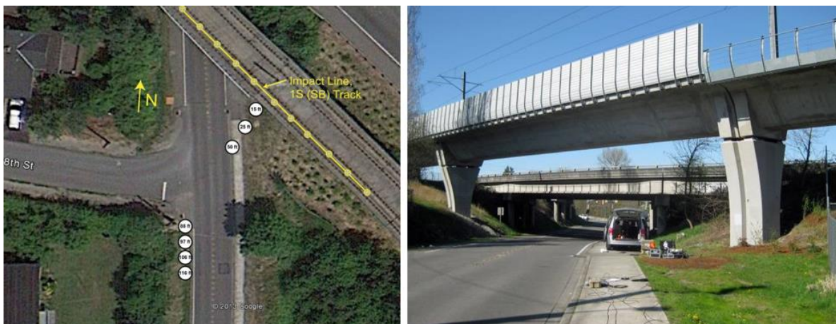
Figure 6: Direct FDL Measurements on Aerial Guideway at Sound Transit, Kinkisharyo LRV
