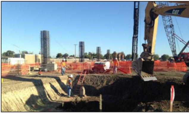
Construction on the pillars that will support the future Berryessa BART Station and elevated trackway.
