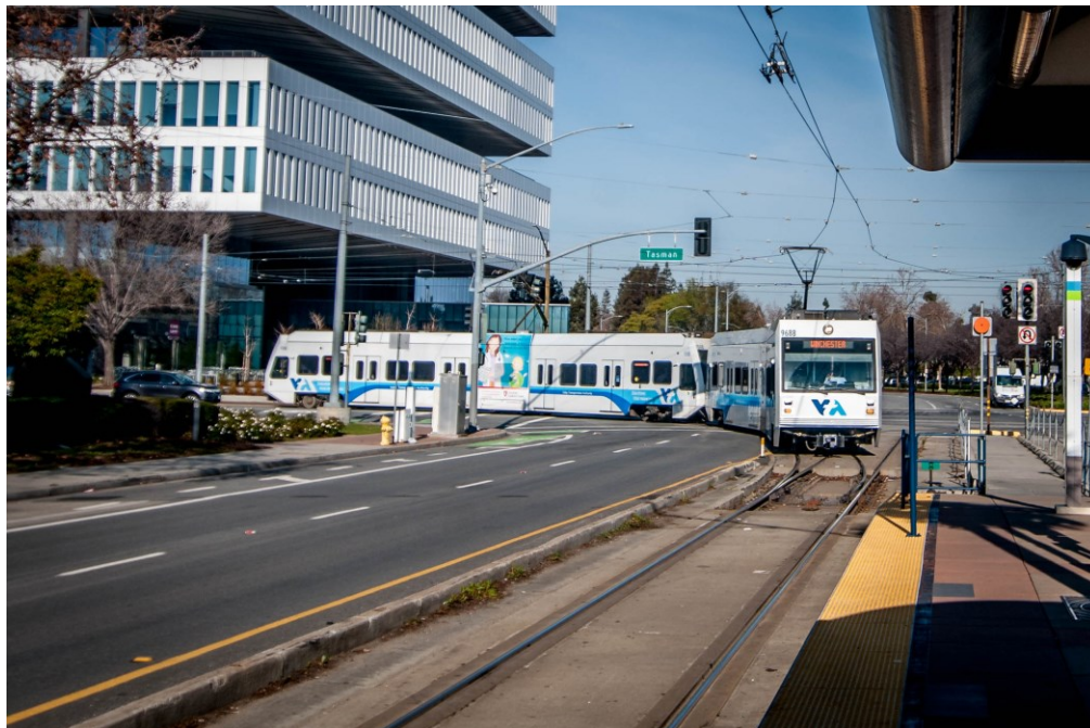
Light Rail Train Approaching Tasman Station
