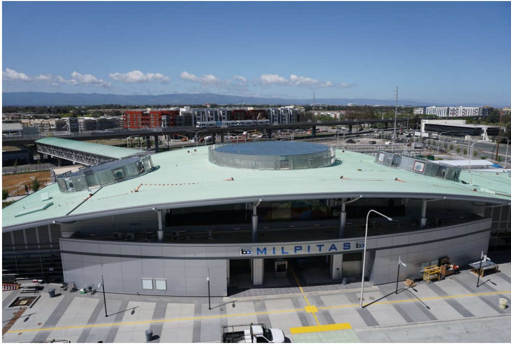
Overhead View of Milpitas BART Station
