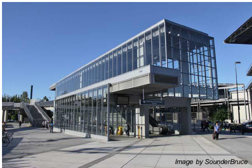
Washington University Station Sound Transit Depth: 95 feet
