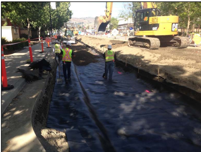
Roadway construction operations on Alum Rock Avenue
