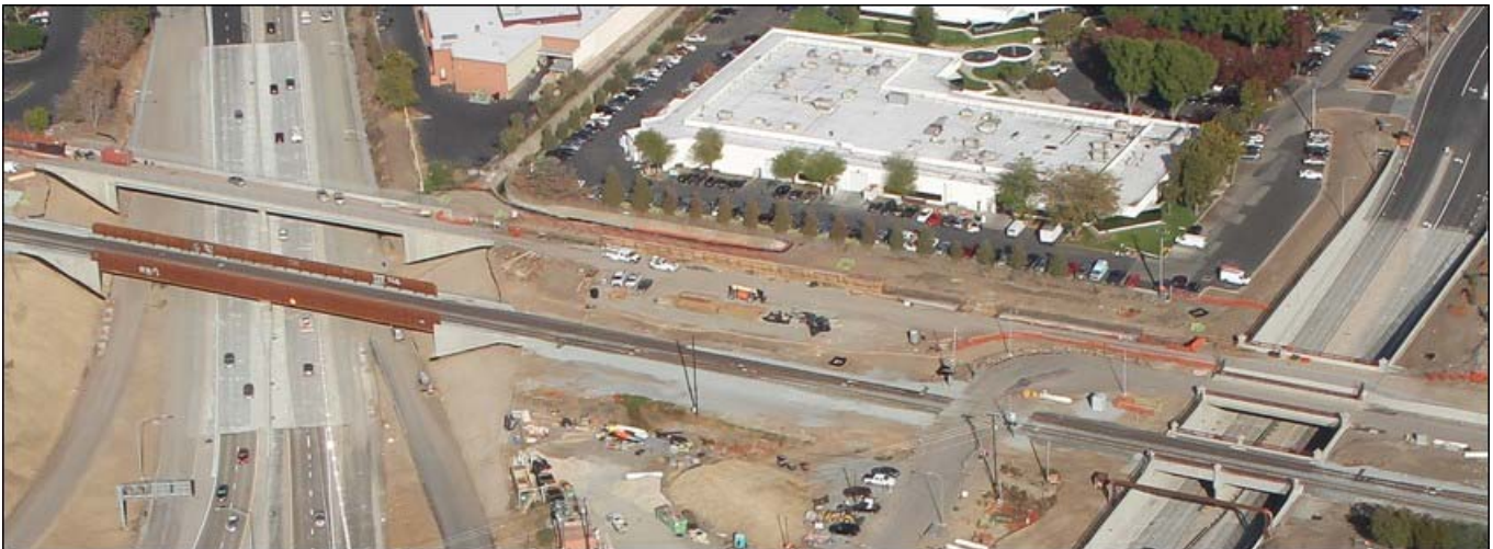
Aerial view of Mission Boulevard (left) and Warren Avenue (right)
