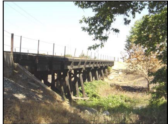
Llagas Creek Bridge
