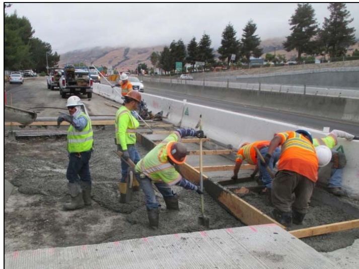
Concrete Placement Along Mission Blvd
