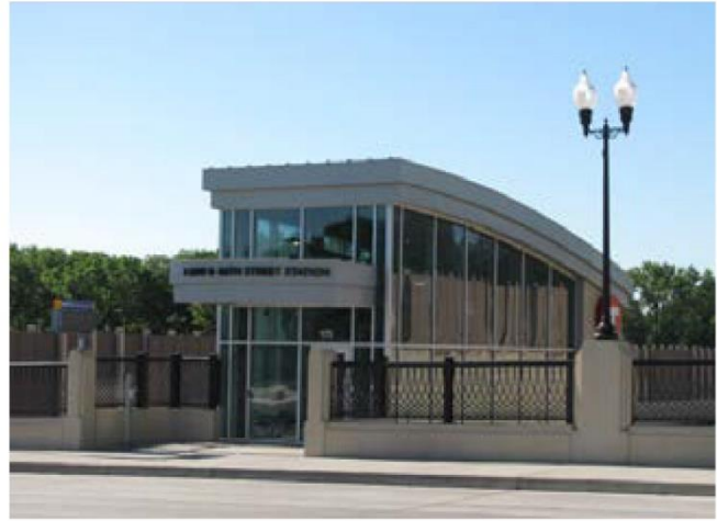
46th: Entrance to BRT Station
