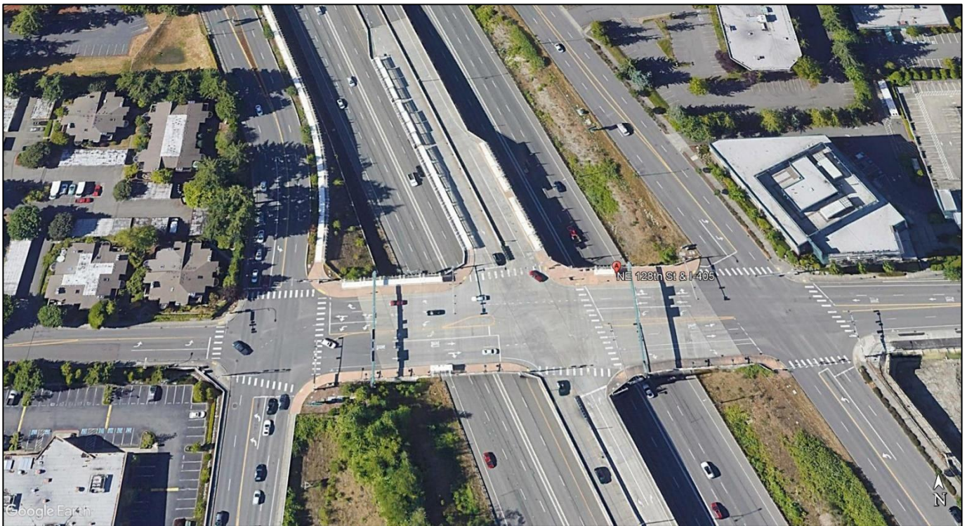
Figure 18 Aerial View of a Median Overpass Station along I-405 at NE 128th Street
