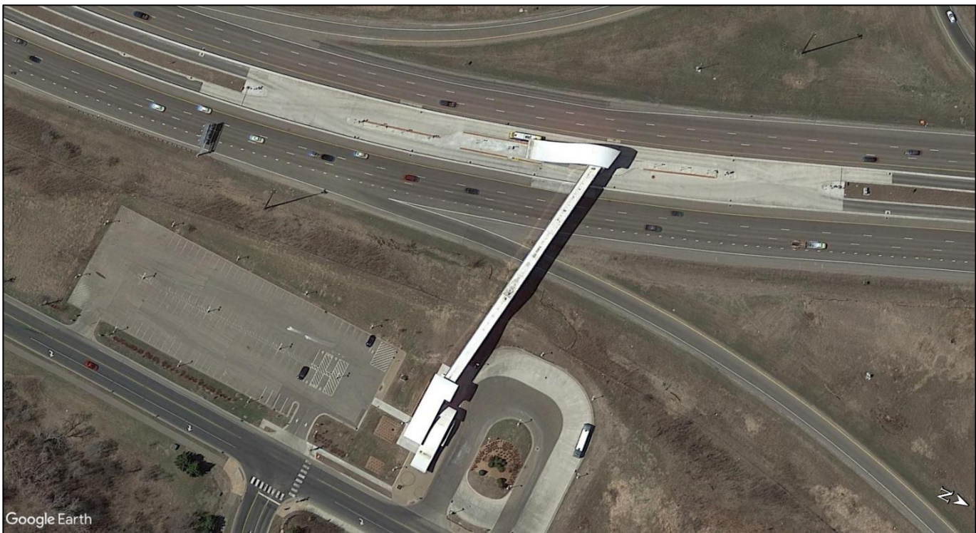
Figure 27 Cedar Grove Transit Station Median Crossover Platform with Pedestrian Overcrossing
