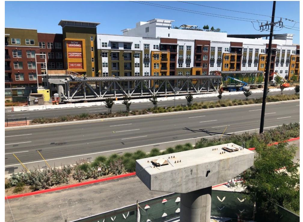
Preparations for Montague Expressway Pedestrian Overcrossing installation
