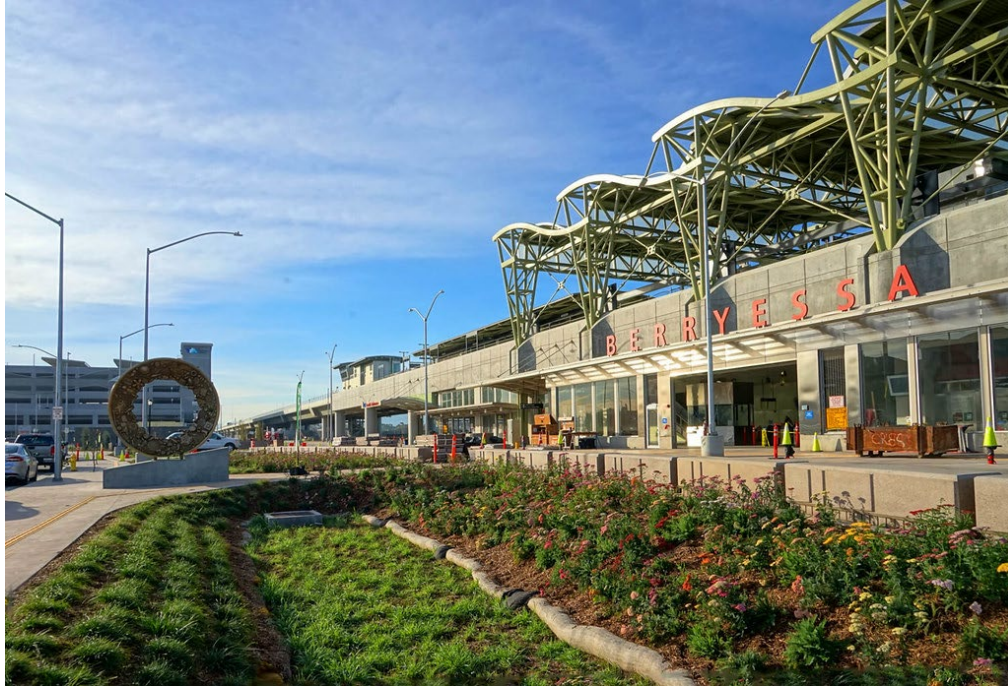
Berryessa BART Station
