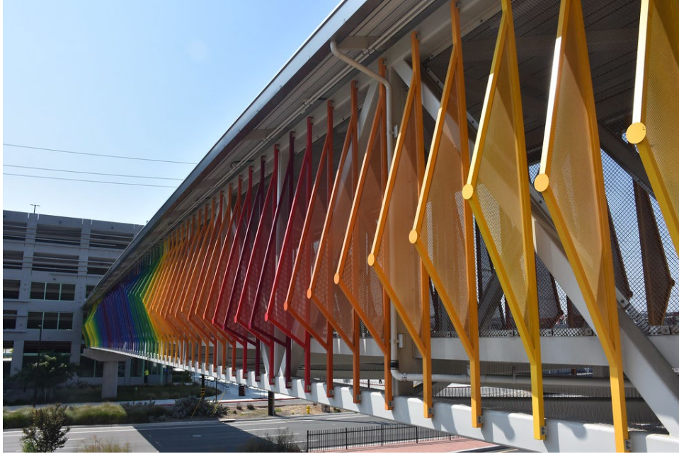
Montague Expressway Pedestrian Overcrossing
