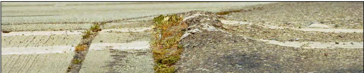
Asphalt bulge at end of bridge deck
