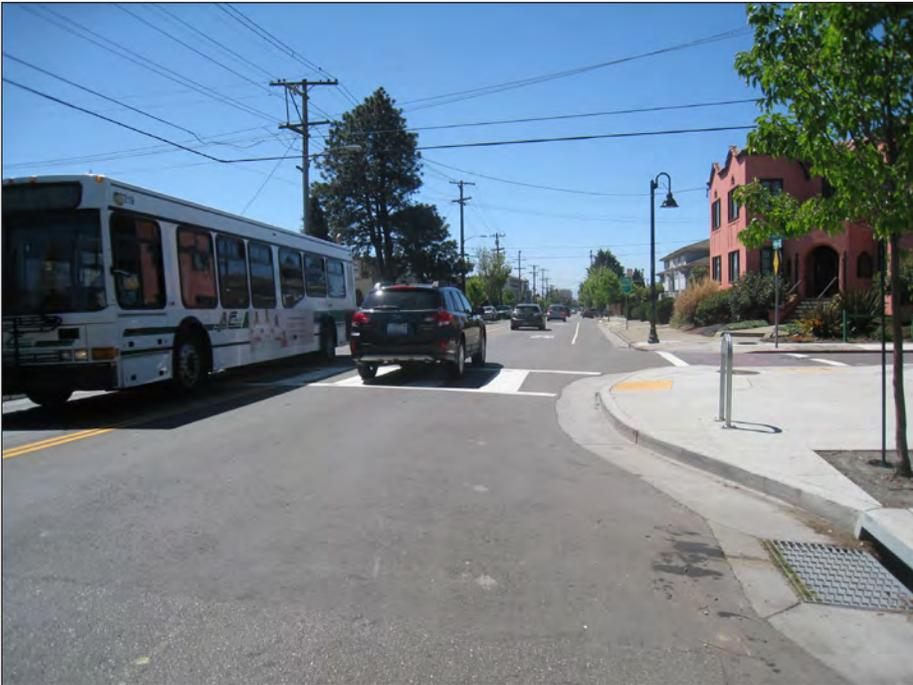
*The wide gutter pan at this bulbout reduces the available smooth obstacle-free roadway width for a cyclist.*
