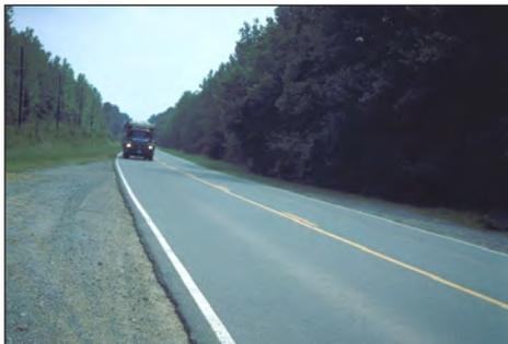
Wide shoulders as in the top photo provide room for cyclists as well as disable motorists; the soft shoulder in the lower photo is adequate for pedestrians in good weather, but is not suitable for cyclists to ride in.
