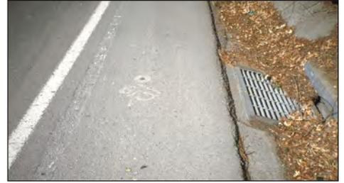
*This drainage grate located off of the shoulder will not force cyclists into the travel lane in order to avoid it.*
