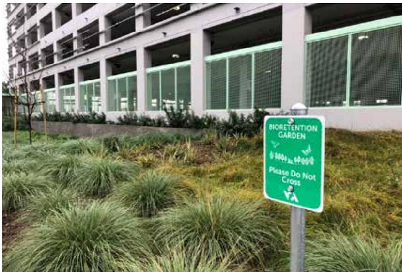
**Figure 15:** Bioretention Basin with Safety Signage
