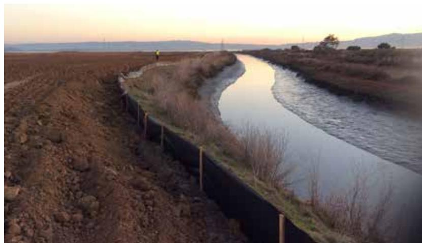
**Figure 5:** Temporary Perimeter Sediment Control with silt fence
