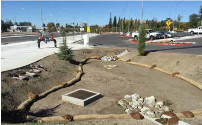
**Figure 6:** Bioretention basin is inadequately protected with only fiber rolls. Note the accumulated sediment filling the rock riprap and discoloring the soil media on the left half of the basin.
