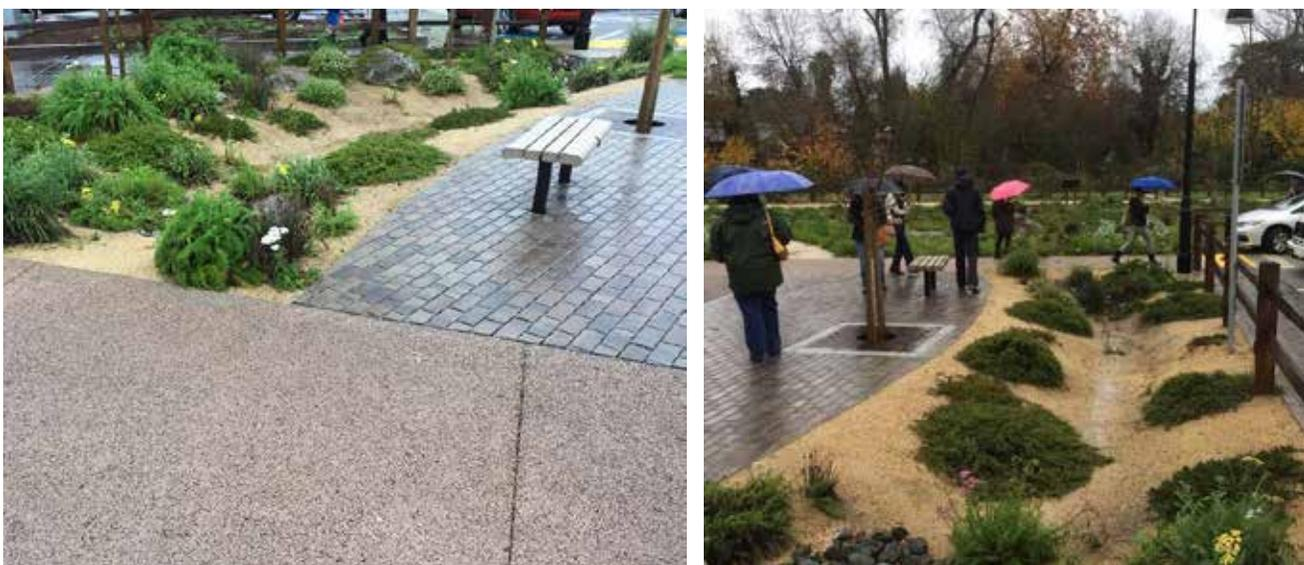
**Figure 10:** Parking Lot with Runoff Reduction Measures
