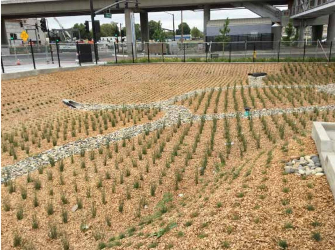
*A guide for the care and maintenance of the SVBX bioretention basins*
