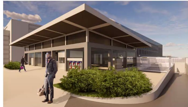
View from Top of Ped Ramp at end of Brokaw Road
