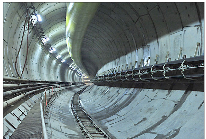
Barcelona's Line 9 Single-Bore Tunnel Source: Sener
