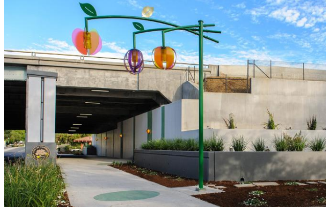
Campbell Ave Portals under State Route 17, Campbell
