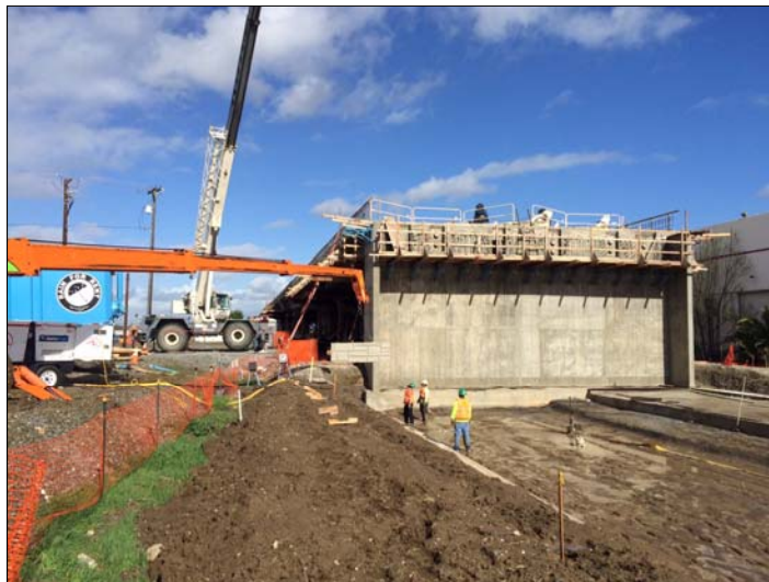
Mechanically Stabilized Earth (MSE) wall construction south of Mabury Road In San Jose
