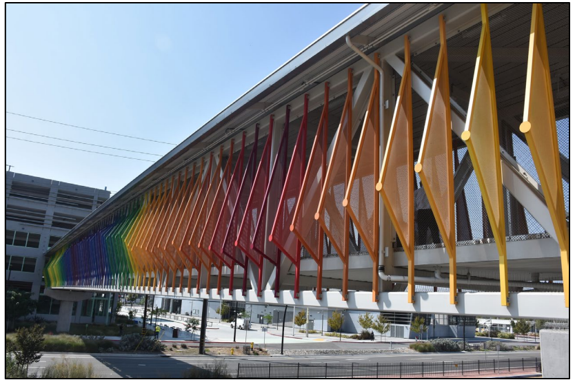
Montague Pedestrian Overcrossing Bridge
