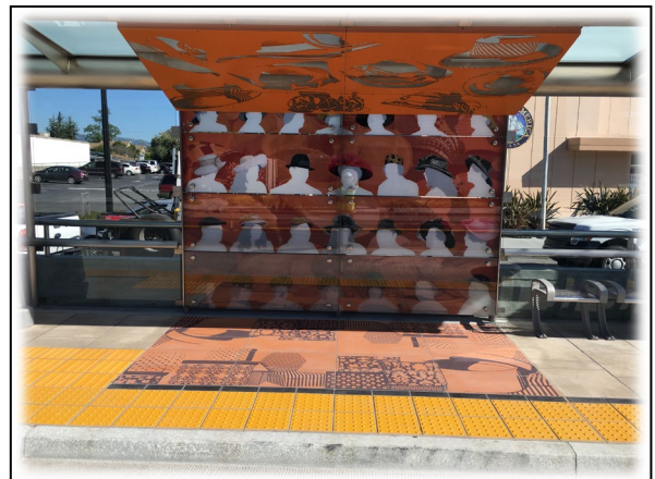
Jackson Street Eastbound BRT Station Shelter
