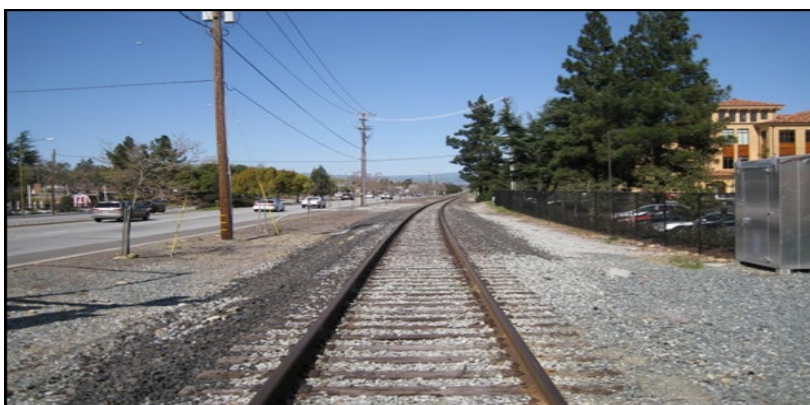
Railroad alignment in Los Gatos, terminus of the Vasona extension
