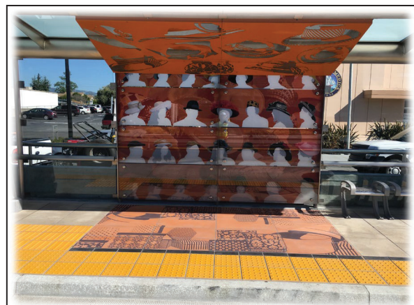
Jackson Street Eastbound BRT Station Shelter
