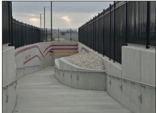
Santa Clara Pedestrian Underpass opened to traffic in June 2017
