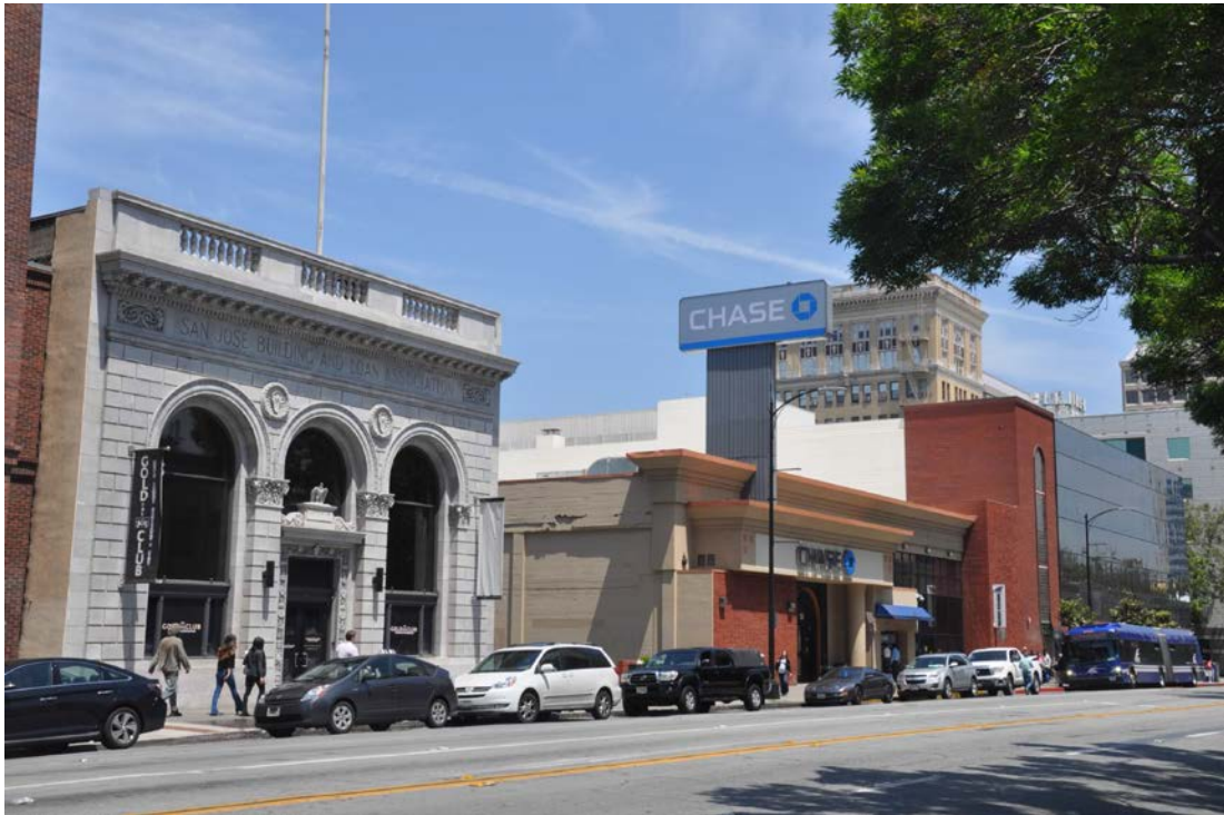
Existing view of Lightson Alley (view to the northeast from Santa Clara Street)
