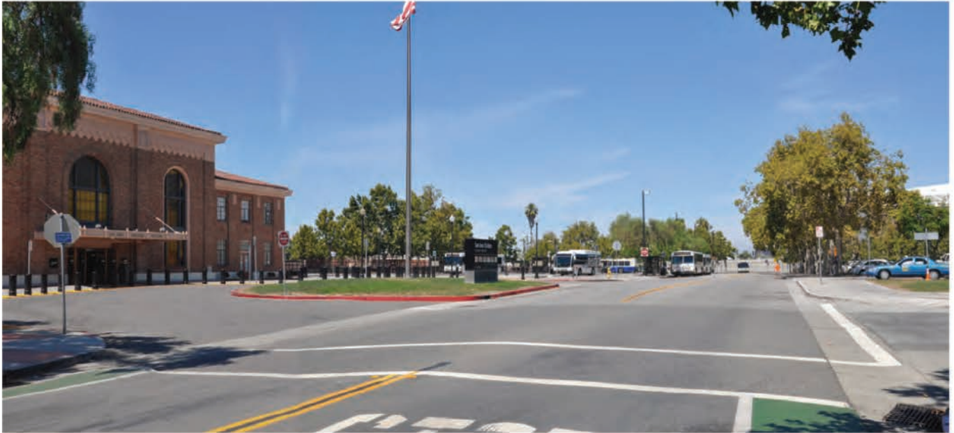
Existing view of the Diridon Caltrain Station (view to the northwest from Cahill Street)
