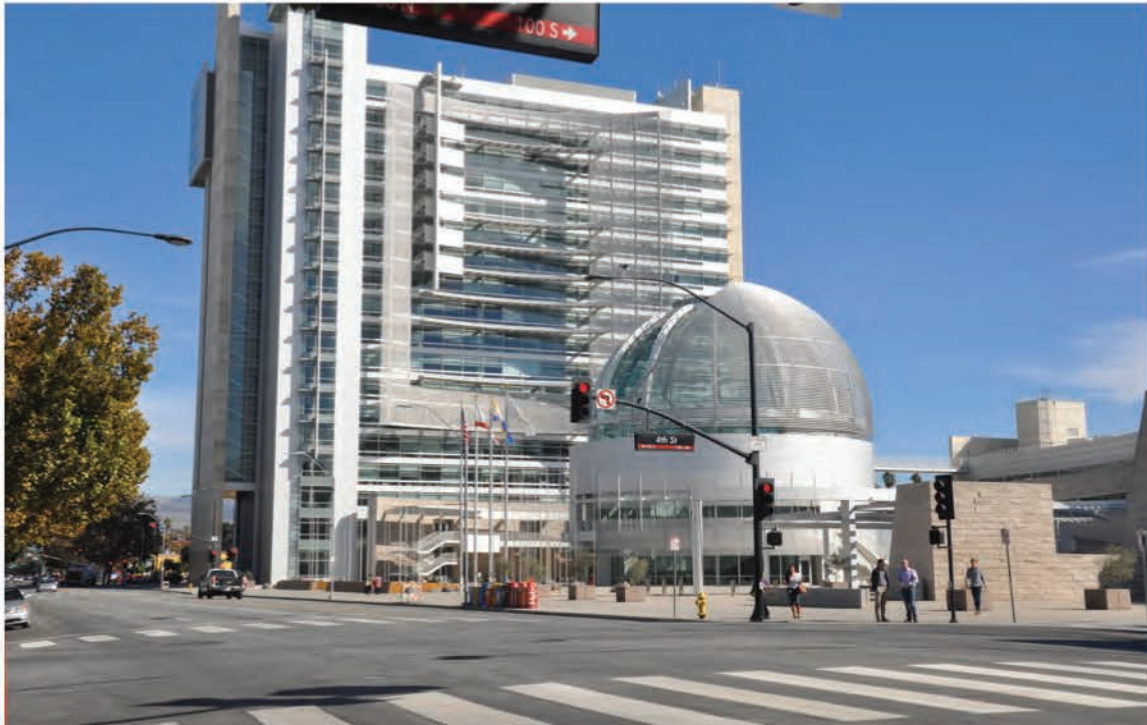
Existing view of City Hall (view to the east from the intersection of East Santa Clara Street and North 4th Street)
