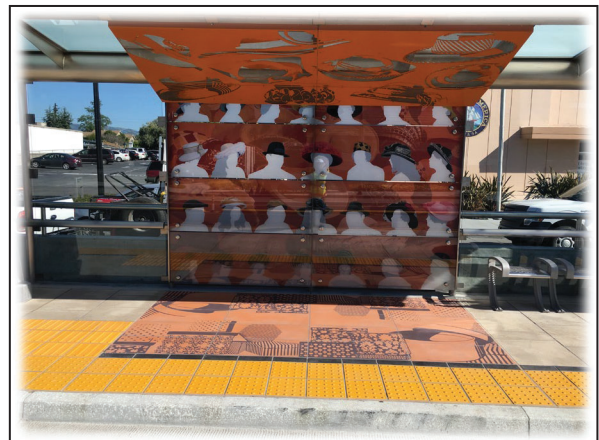
Jackson Street Eastbound BRT Station Shelter
