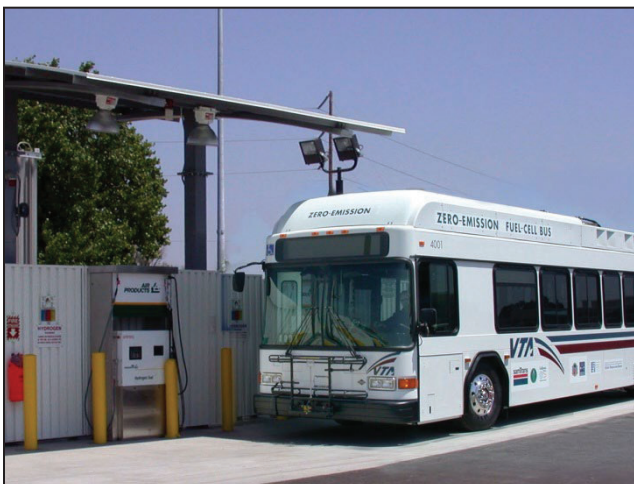
ZEB at Fueling Station
