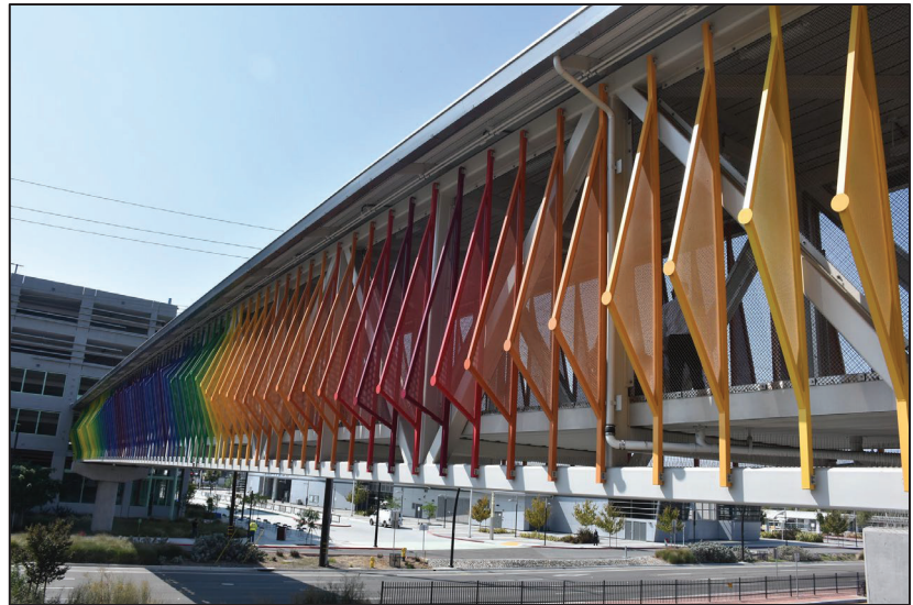
Montague Pedestrian Overcrossing Bridge
