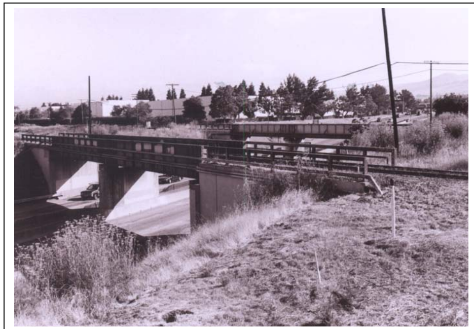
Figure 31. Mission Boulevard Bridges (Bridge #33-183, foreground, and #33-184, background).
