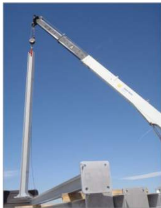
On/off-track crane for installation
