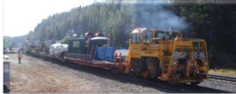
DrillTech on track foundation train
