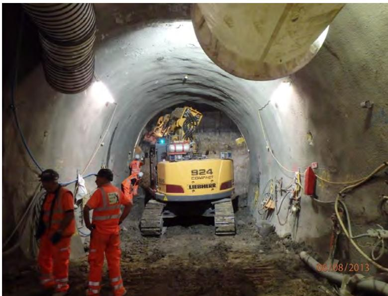
**Figure 5.** Exposed tunnel face during top heading excavation of PL2RC with the Liebherr 924 excavator.
