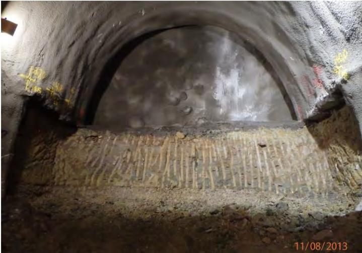
**Figure 22.** Exposed Bench during the construction of PL2RC. Strip reinforcement was not used for the formation of the radial joints, to ease the forthcoming passage of the Westbound TBM.
