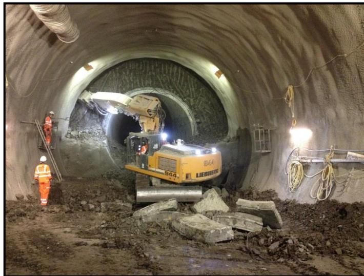
**Figure 4 – Sequentially Excavated Sprayed Concrete Tunnel**
