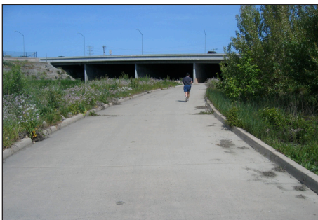
Guadalupe River Trail, with its numerous undercrossings, is essentially a bicycle "freeway".
