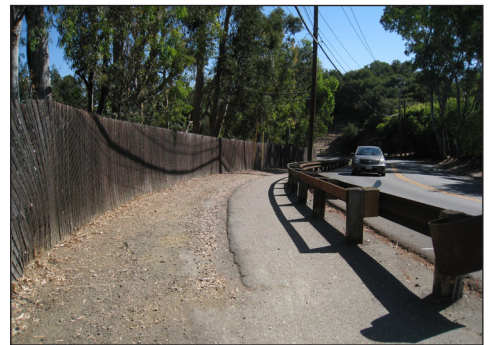
This roadside path in Los Altos Hills is separated from the roadway by a guard rail within the horizontal curve.
