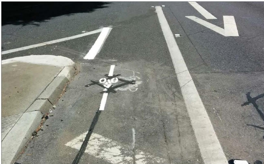
b. View of a bike detector embedded in a bike slot. The purpose of a bike detector is to detect a bicyclist approaching an intersection and communicate with the traffic signal cabinet to provide enough time for cyclists to safely cross an intersection.
